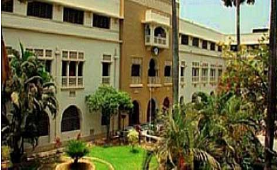
Indo-Saracenic architecture prominent in the college main building and garden
